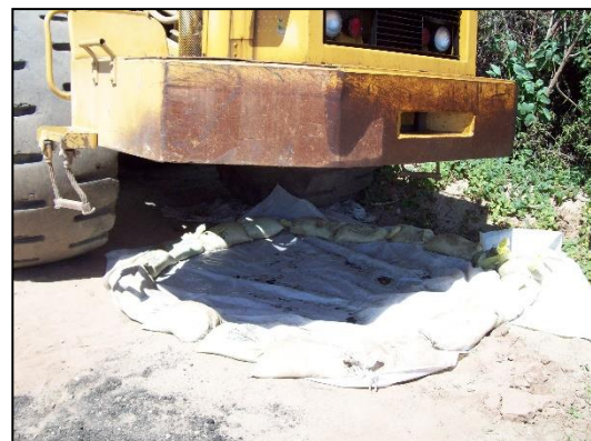
Gravel bags and tarps offer effective containment of possible leaks.
