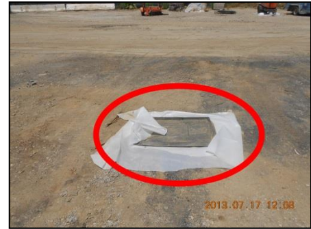
Basic drip pan for collecting leaks
