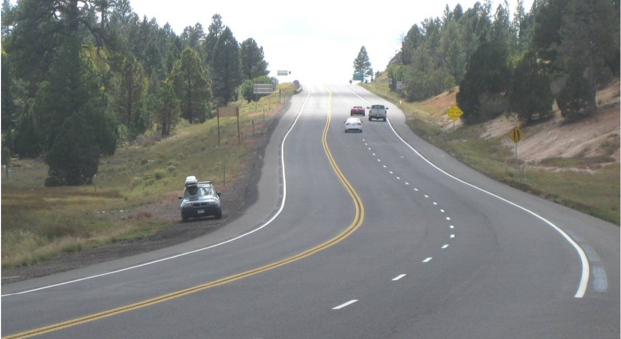
Passing Lane SB 3 ending prior to crest of hill.
