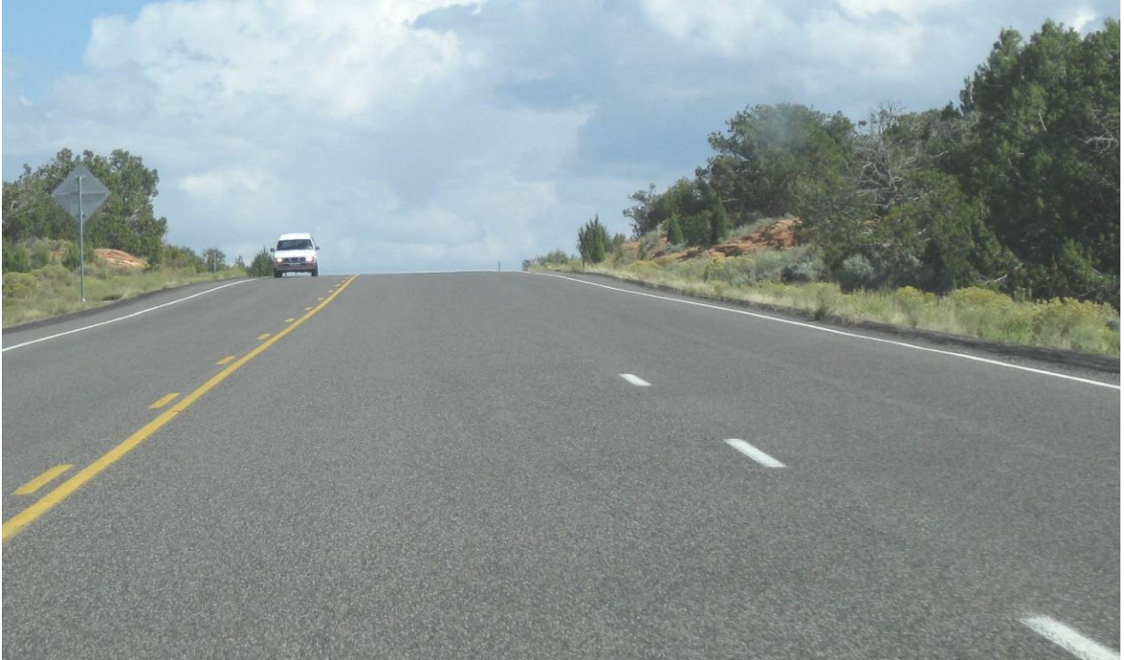
Passing Lane SB 5 ending prior to crest of hill.
