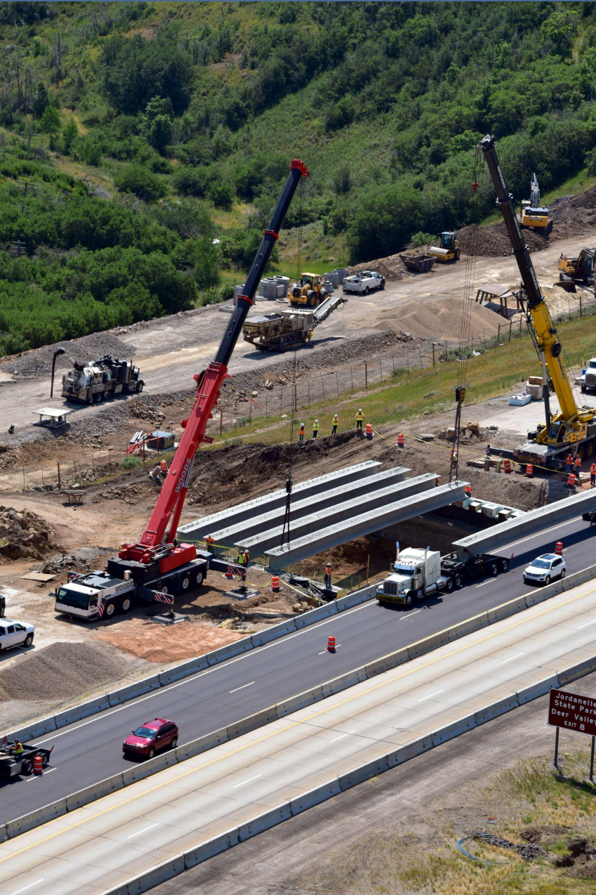
Crews placing bridge girders at north portal during summer 2020
